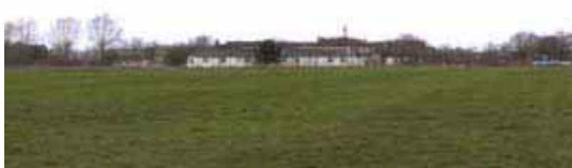
Looking west to 'White Huts' from Blackburn Road (east boundary of site).
